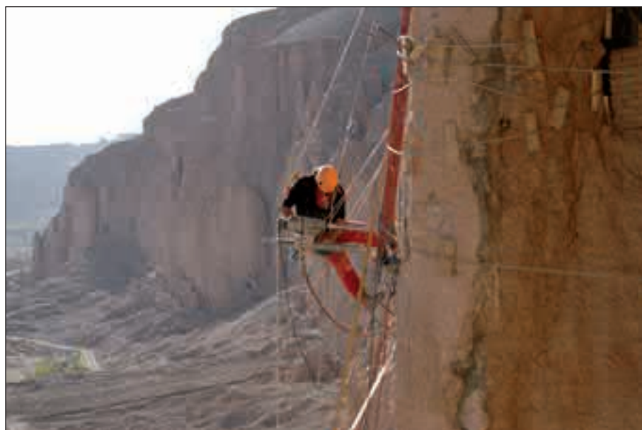
Fig. 29. Drilling for the setting of nails ▷
