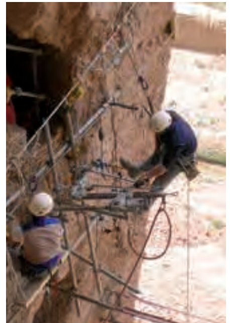
△ Fig. 16 Installation of temporary struts. During the installation the strut is fixed at the top of the cliff, in the safe zone
