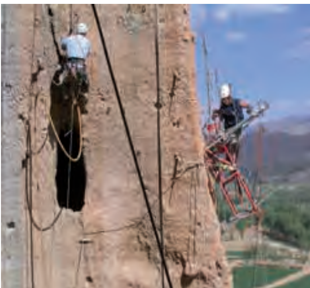
▽ Fig. 21 Detail of execution of nails from inside the caves by means of a small rotary machine and a diamond head
