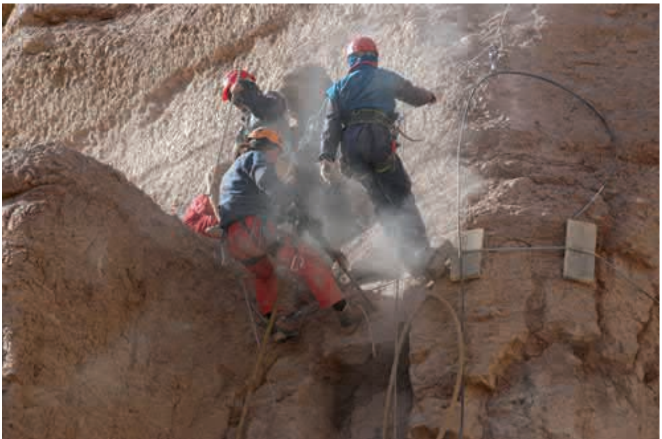
Fig. 36. Drilling the lower part of the niche
