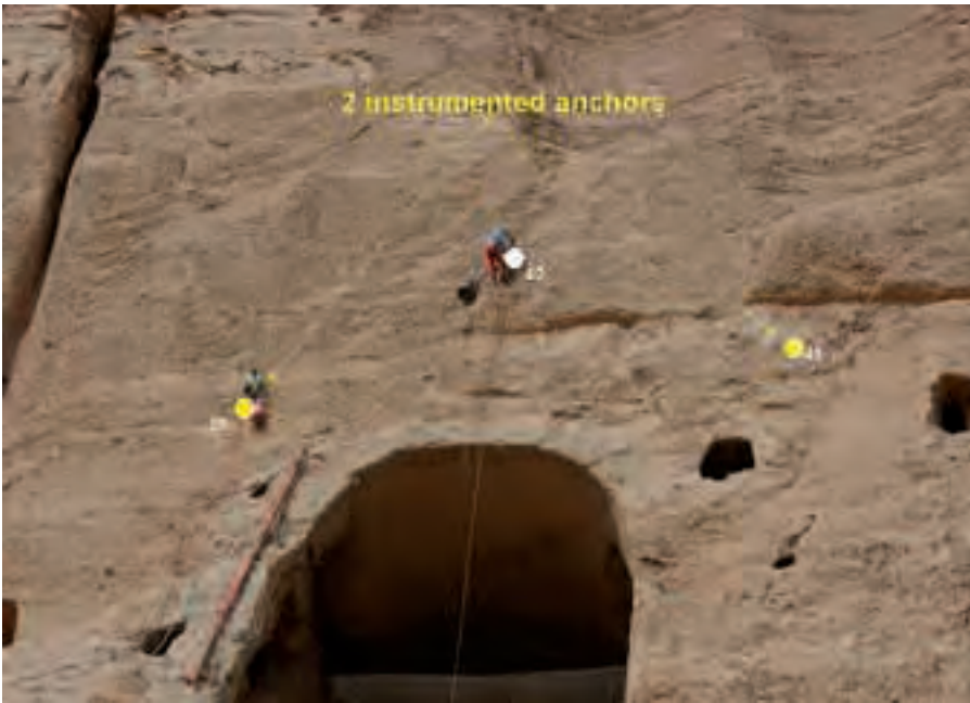
◁ Fig. 30. Position of anchors on top of the niche. The yellow ones are monitored with 10 strain gauges
