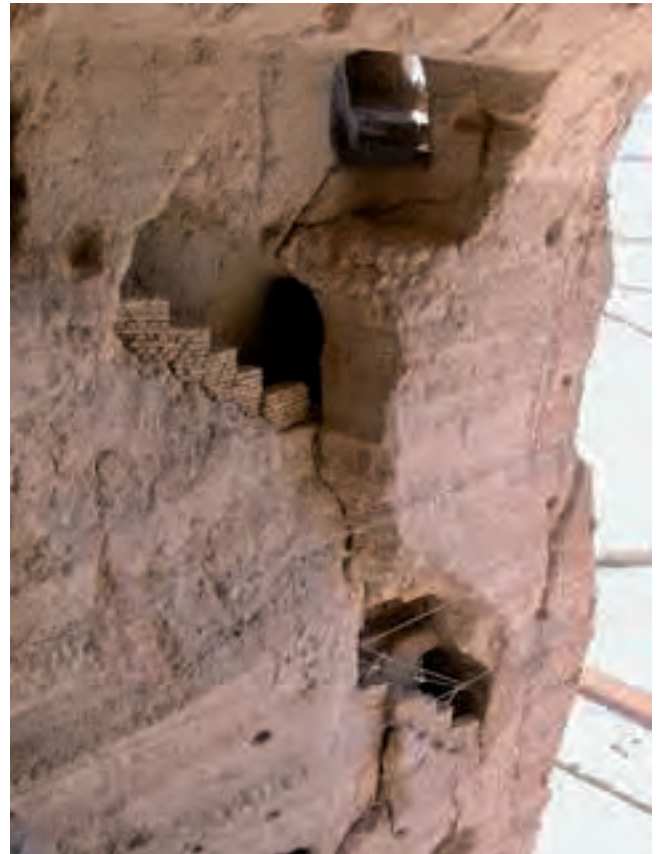
Fig. 13. The temporary beam (left) and steel rope (right) for the temporary support of the upper eastern part of the Eastern Buddha
