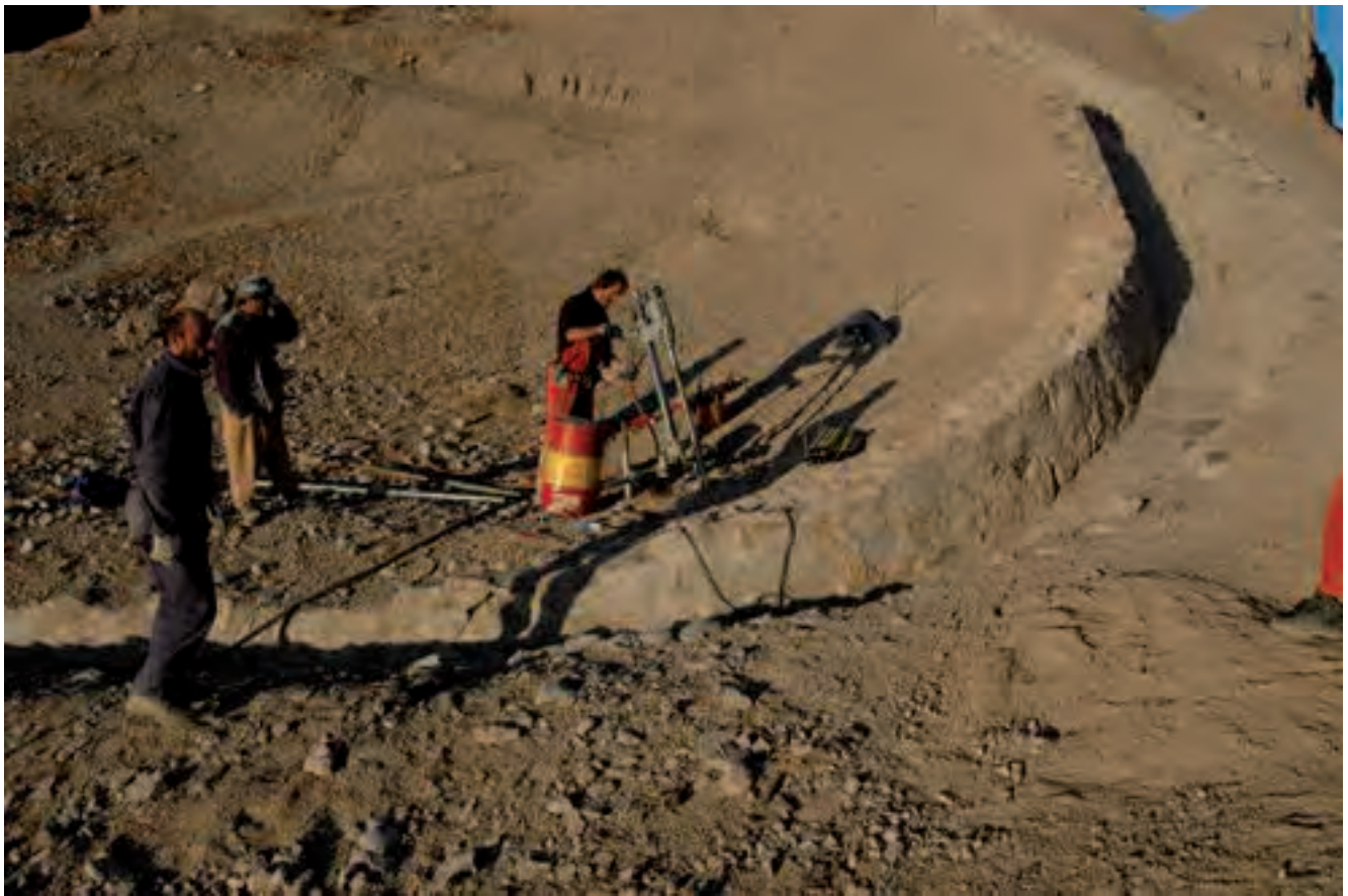
Fig. 35. Detail of the grouting from the top of the cliff
