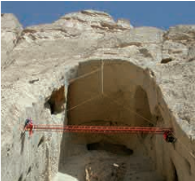
△ Fig. 16 Installation of temporary struts. During the installation the strut is fixed at the top of the cliff, in the safe zone
