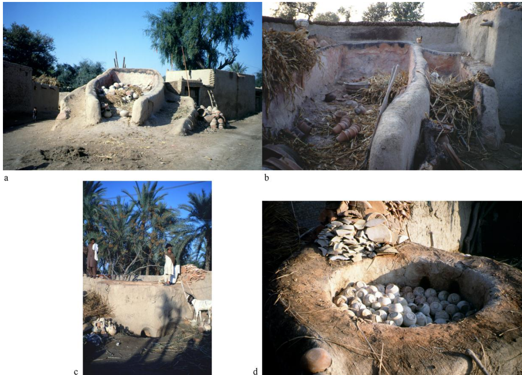
Figure 5. Range of pottery kilns (see also the simple kiln for firing thaibi, in Figure 3b): (a) a communal horse-shoe shaped sloping kiln (9.5 m long by 2.8 m wide, height ranging from 0.6 to 1.5 m) located in an open space in the village of Gandi Khan Khel; (b) double kiln in the courtyard of Gul Nawaz (village Nurar), the larger one (7.8 x 3.0 m; from 0.4-0.8 m high) is for firing a range of pots, while the smaller one (3.8 x 2.0 m; from 0 – 0.45 m high) is for firing thaibi; (c) circular updraft kiln (outer diameter 3.5 m, inner diameter 2.1 m, outside height 1.2 m) in the courtyard of Said Ghani (village Shabaq Azmat Khel); (d) Said Ghani's updraft kiln loaded with water pots.
