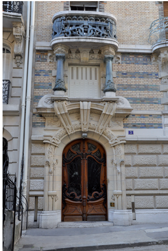
Fig. 5. Architectural photograph, detail of the entrance doorway, 3 square Rapp, Paris (Jules Aimé Lavirotte, Alexandre Bigot, 1899); CC BY-SA 3.0 Wikimedia, available online: http://upload.wikimedia.org/wikipedia/commons/2/29/Immeuble_3_square_Rapp_Paris_7e_-_Entr%C3%A9e.jpg , accessed 4 September 2014
