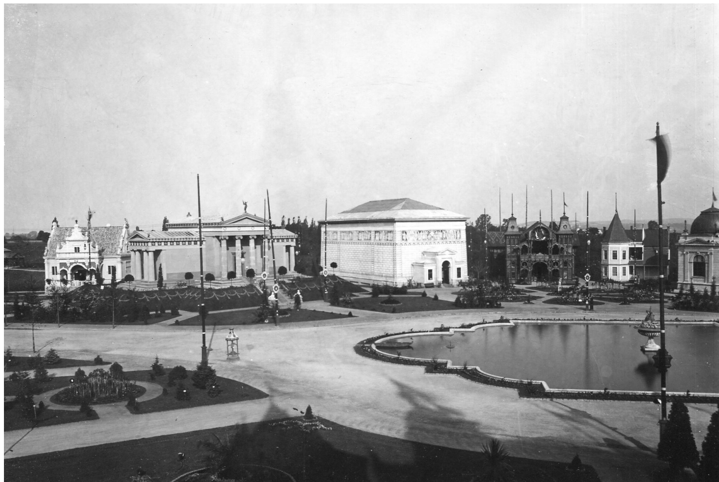
6. The main square of the Land Exhibition (Western side). The Pavilion of architecture, Matejko's Mausoleum, the pavilion of the city of Lviv. The collection of Kotlobulatov's family, Urban Media Archive of the Center for Urban History of East-Central Europe
