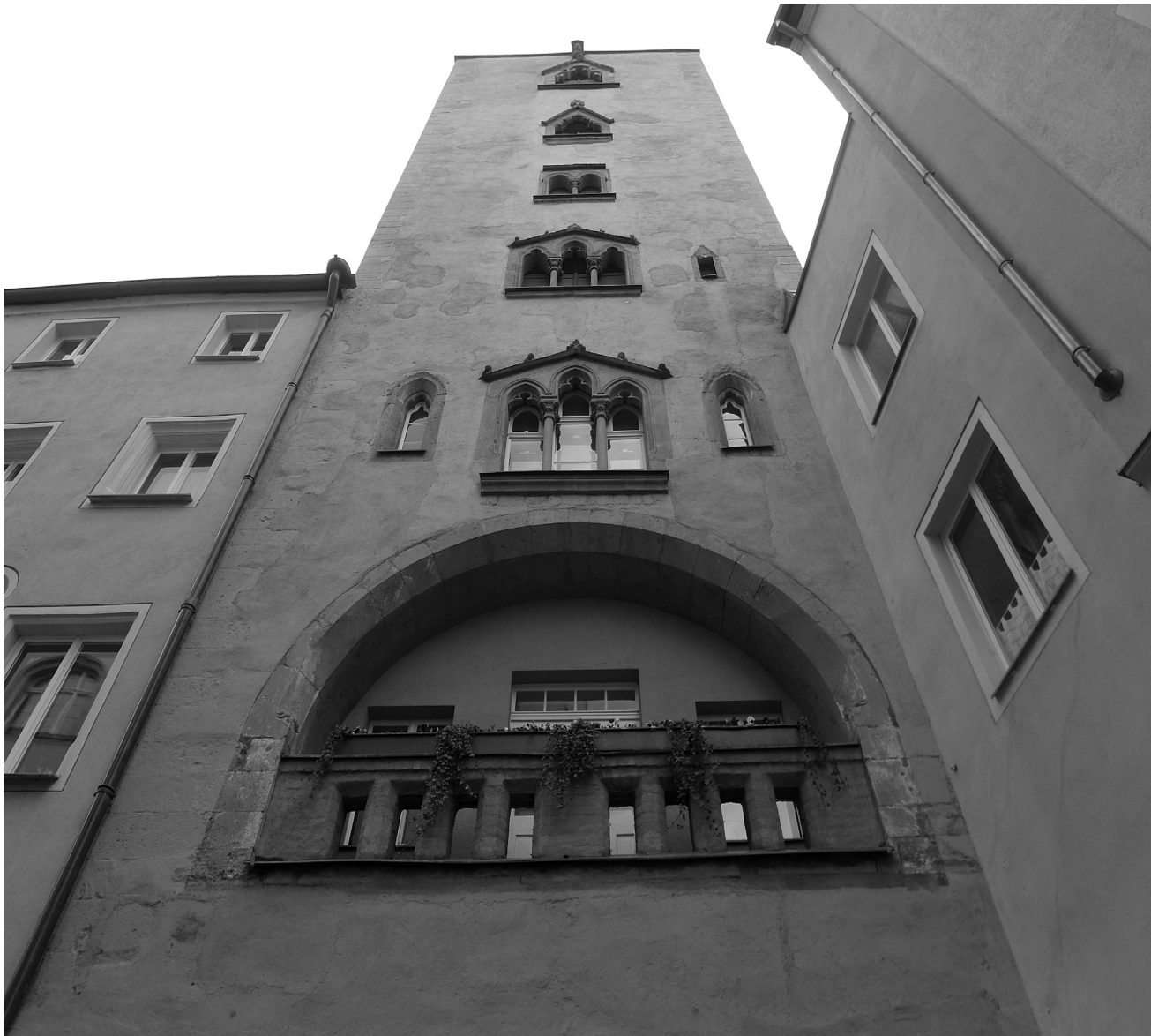
13. Baumburger Turm, tower with loggia, Regensburg. Photo: R. Eysymontt
