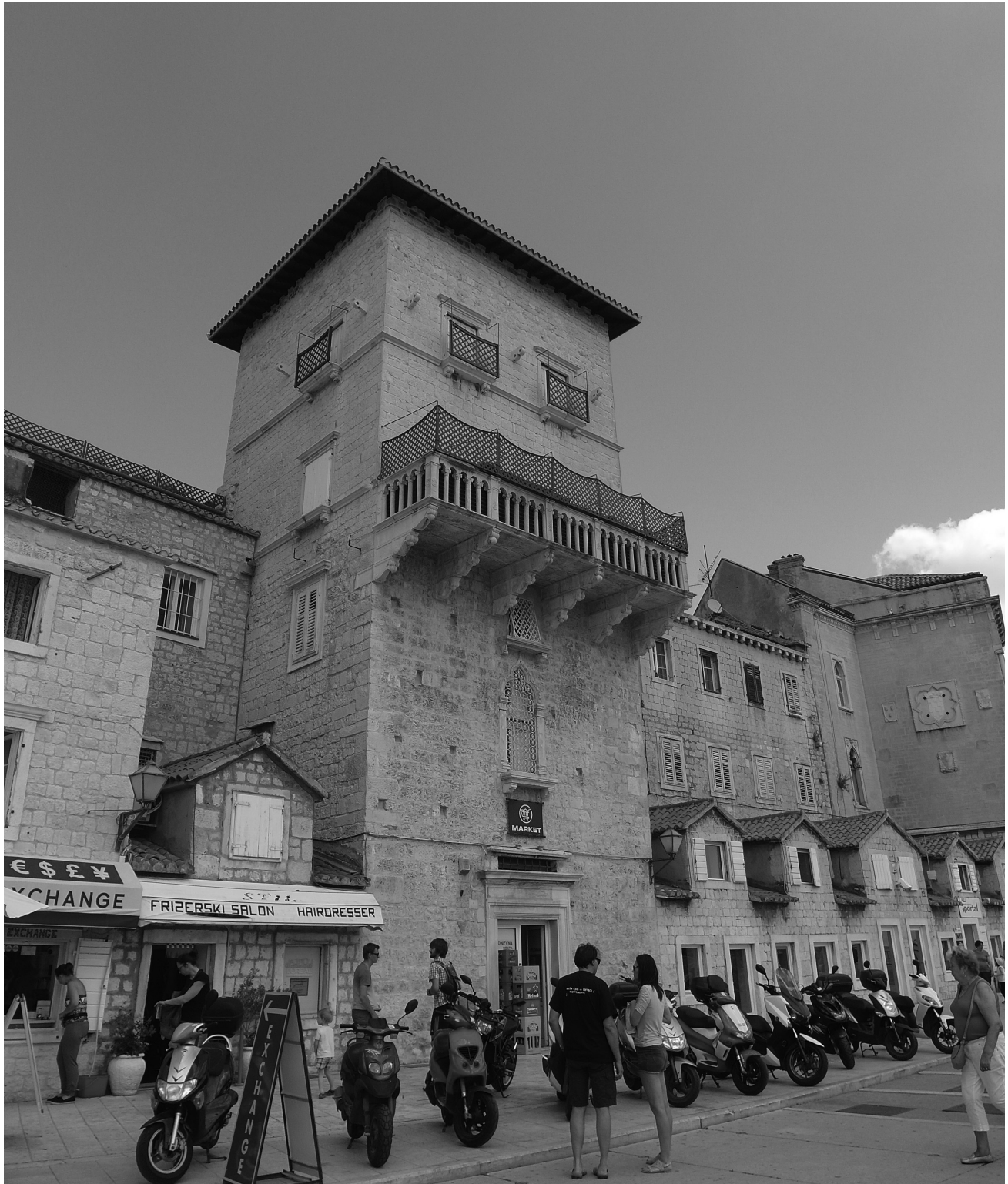
9. Vitturi tower, Trogir. Photo: R. Eysymontt
