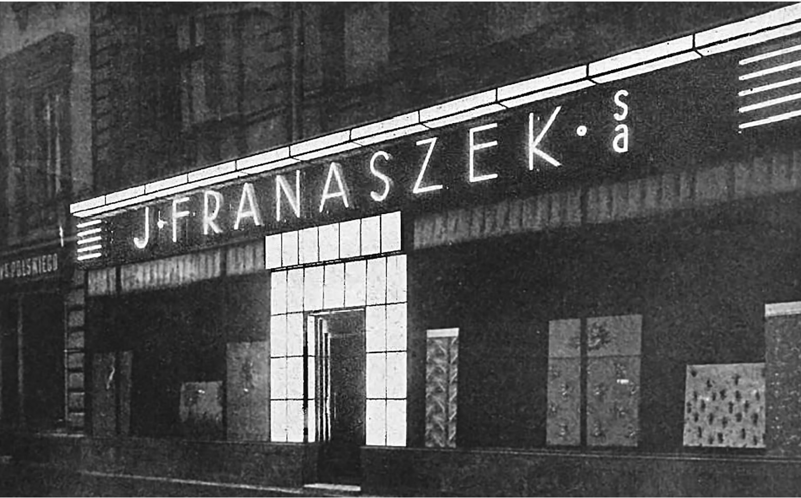
fig. 7 S. Siennicki, shop window of "J. Franaszek S.A." in Jerusalem Avenue 33 in Warsaw, 1931. Photo from: "Przegląd Budowlany" 1931, no. 6/7, pp. unnumbered
