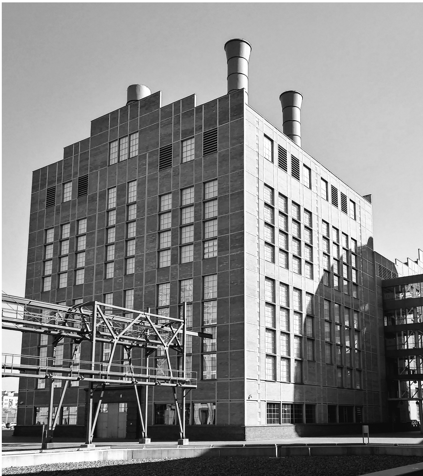
— fig. 2 New Central Unit at the EC1 power plant in Łódź, 1929–1930. Photo: F. Burno
