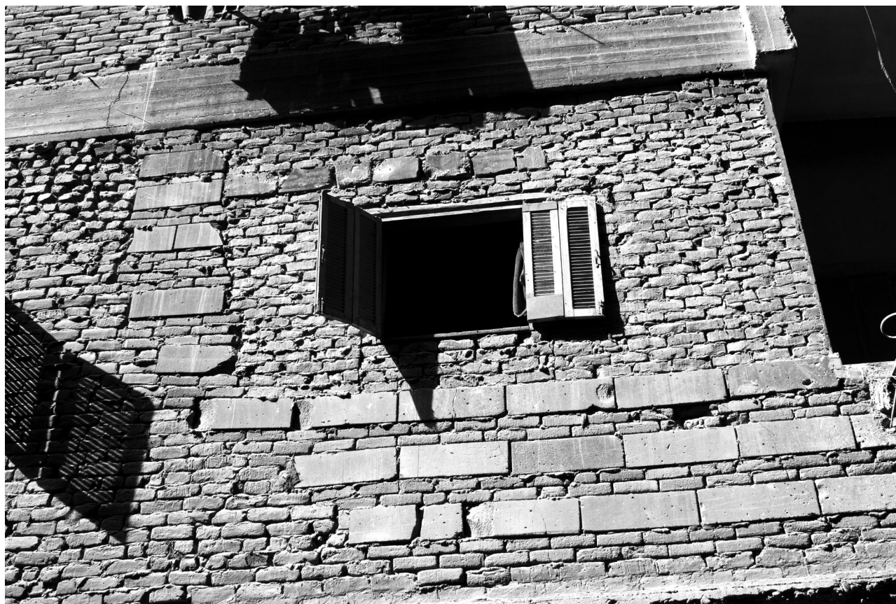
fig. 8 Adobe brick facade, Garbage City, Cairo, Egypt 2019. Photo: K. Wiącek
