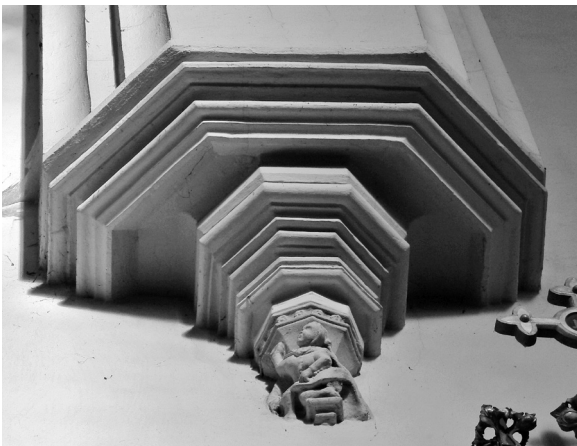
14. The corbel of the inter-naval arcade in the St. John the Evangelist Church in Paczków, before 1389. Photo: R. Kaczmarek
