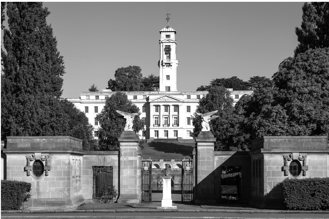
8-9. Clare Hartwell, Nikolaus Pevsner, Elizabeth Williamson, Buildings of England: Nottinghamshire , London 2020, Plate 100: Trent Building, University of Nottingham (1928). Photo: M. Hamilton Knight
