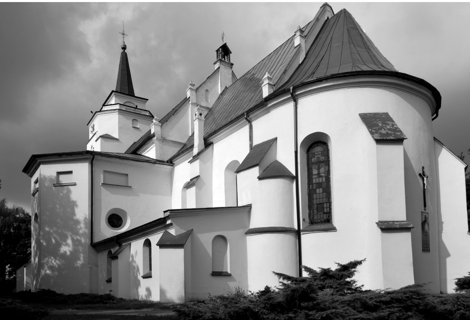
7. Kowal, parish church. View from the south-east. Photo: W. Miedziak
