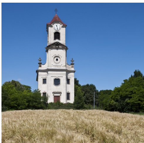
6 Stranzendorf, parish church of SS Peter and Paul (1733), main facade with an incorporated belfry (photo: P. Mofardin)
