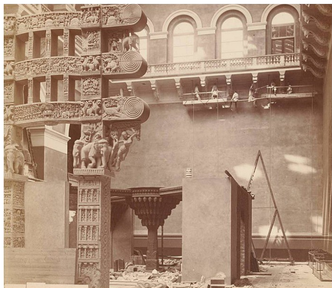
8 Installation of the casts of the Sanchi gateway and the corbelled pillar from Fatehpur Sikri in the Architectural Courts of the South Kensington Museum, London, in 1872 (courtesy: V&A Archive, London)
