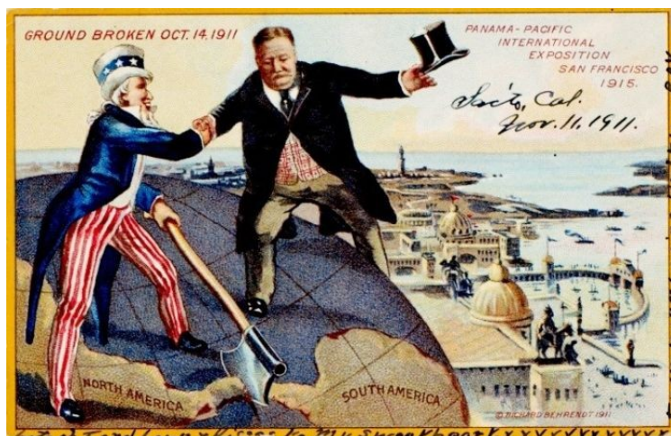
5 "Ground Broken Oct. 14, 1911. Panama-Pacific International Exposition, San Francisco, 1915", postcard. San Francisco History Center at San Francisco Public Library (photo: SFPL, San Francisco, CA)
