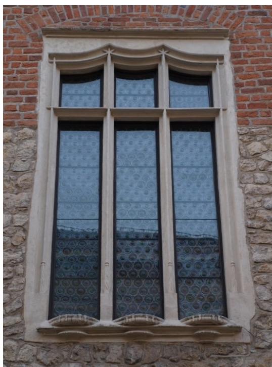
8 Collegium Maius of the Jagiellonian University, Cracow, one of the curtain arch windows in the northern wall of the Aula , 1507–1510 (photo: author)
