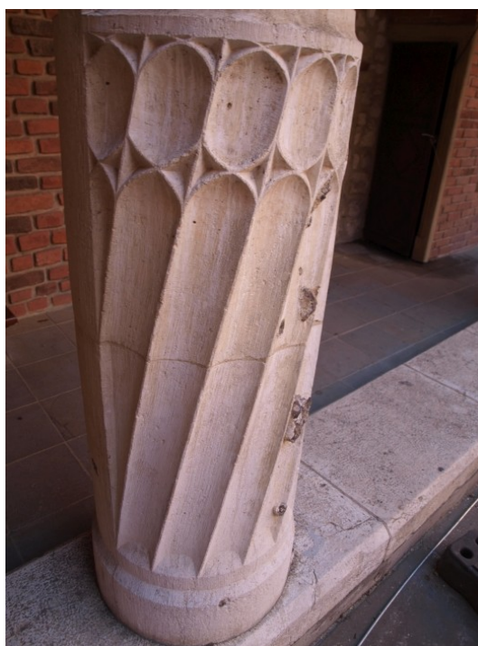
5 Collegium Maius of the Jagiellonian University, Cracow, cloister, one of the pillars with spiral flutings, after 1493 (photo: author)
