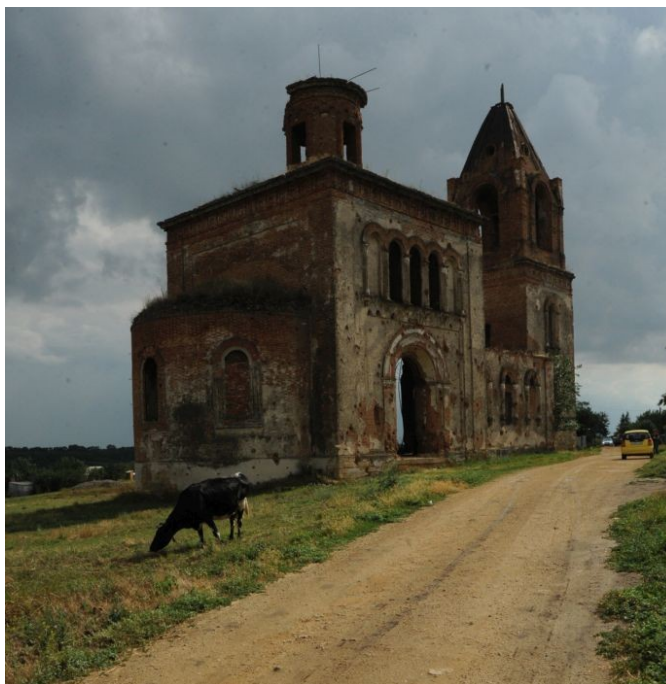
8 Village of Sultan Saly, church of Surb Gevorg, mid-19th century, architect unknown. General view from the North-East (photograph: A. Kazaryan, 2017)
