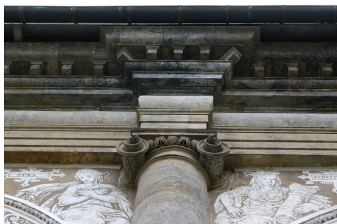
11 The Great Ball Game Hall, Prague Castle, detail with painted decoration of the entablature and the upper part of a column, after the renovation in 2018–2019 (photo © Sylva Dobalová, 2019)
