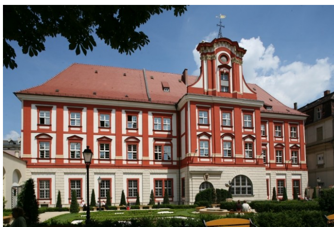
8 Former Monastery of the Knights of the Cross with the Red Star, Wrocław, 1675-1715, design: Jean-Baptiste Mathey (photograph © Martin Mádl)
