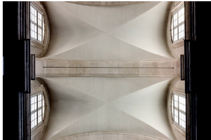
14 The Cathedral, Dubrovnik, cross vaulting in the main nave constructed according to the design of Tommaso Napoli (photo: P. Mofardin)
