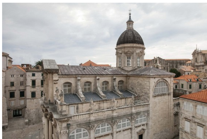
17 The Cathedral, Dubrovnik, view of the terraces and the upper area with buttresses for the vaulting, made according to the design by Tommaso Napoli (photo: P. Mofardin)
