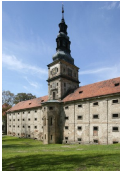
25 Jean Baptiste Mathey, Plasy, granary of the former Cistercian monastery, 1685-1686, photo: Martin Mádl
