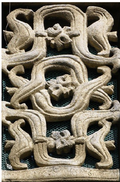
3 Jerzy Jarnuszkiewicz & Bohdan Lachert, rubble-concrete grid at 8 Katowicka Street in Warsaw, 1946. Photograph by the author
