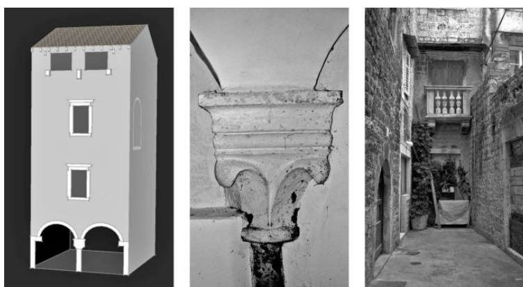
11 Remodelling of the Andreis Tower, Trogir (fig. 3, no. 1): a) southeastern façade with the mid-14 th c. porch and the 17 th c. windows and loggia, and northeastern façade with a Romanesque door that used to connect the tower and the main house on the second floor level; b) porch capital; c) northwestern façade with 18 th c. balcony (© Ana Plosnić Škarić)
