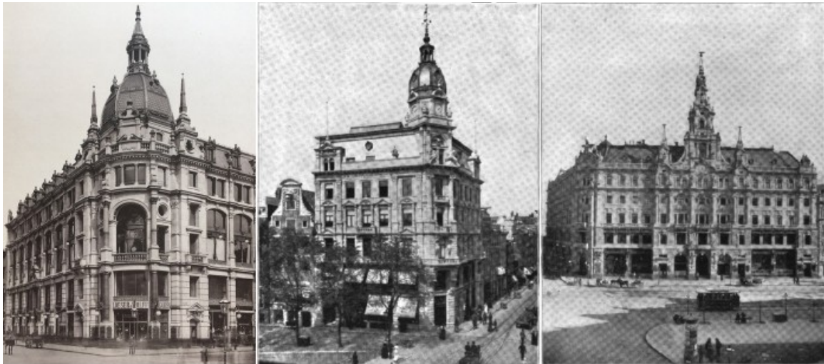
2 a) Equitable Life Building, Berlin (reprod. from: Architektur der Gegenwart , vol. 2, pl. 32) | b) New York Life Building, Amsterdam | c) New York Life Building, Budapest (reprod. from: Hudnut 1895, 213, 219)
