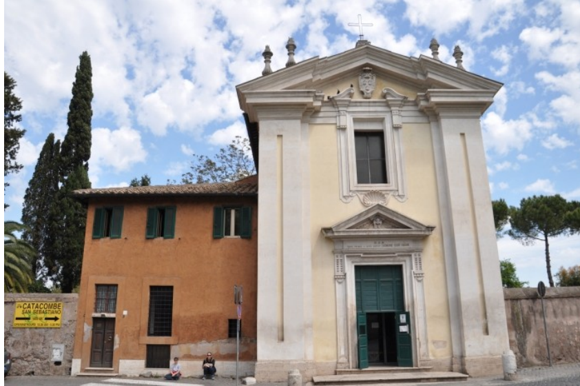
4 Church of Santa Maria in Palmis, south-east of Rome, at the Appian Way, front (photo: A. Bacciolo)
