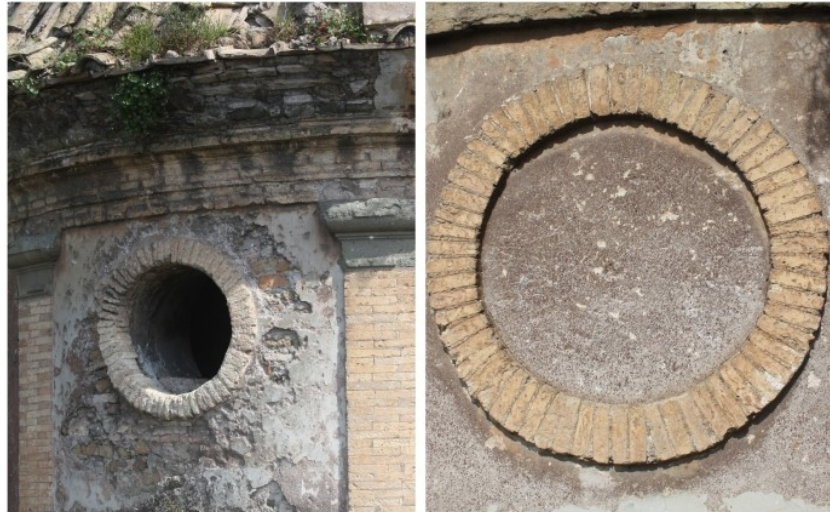
13 Oratory of Domine Quo Vadis, oculi and pilaster shafts (photo: A. Bacciolo)
