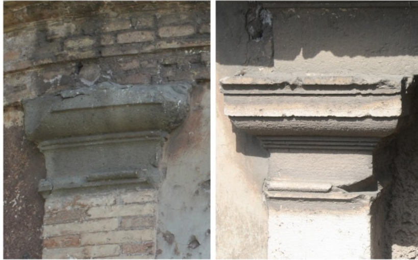
9 Pilaster capitals: (left) Oratory of Domine Quo Vadis, (right) Bramante, Tempietto in San Pietro in Montorio (photos: A. Bacciolo)
