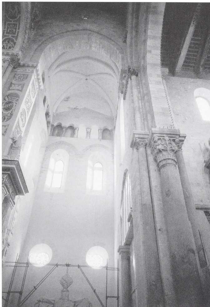
21. Cefalù, cathedral, view into the southern transept with ribbed cross vault
