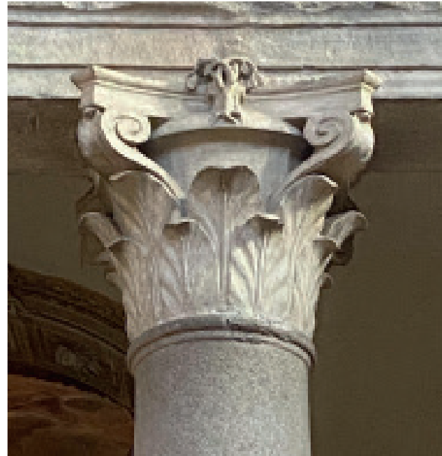
28 Rome, Santa Prassede, nave capitals, antique restuccoed with inverse volutes, 1594/1605 (photo author)
