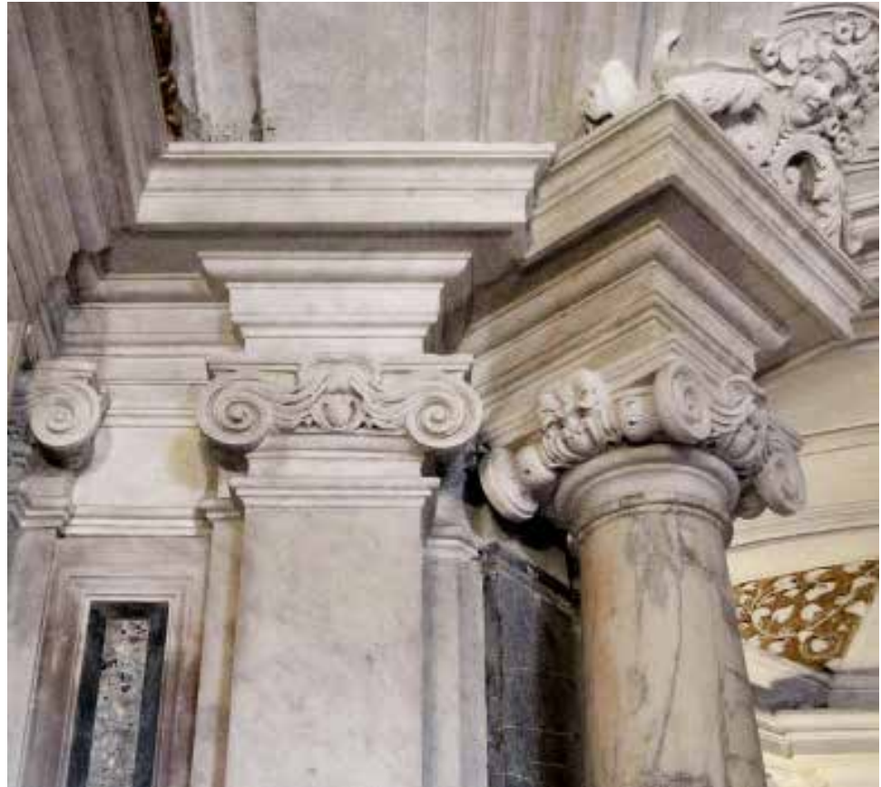
1 Pietro da Cortona, Detail of Ionic pilaster and column of the confessio, executed by Luca Berrettini, 1664. Rome, Santi Luca e Martina (Photo author)
