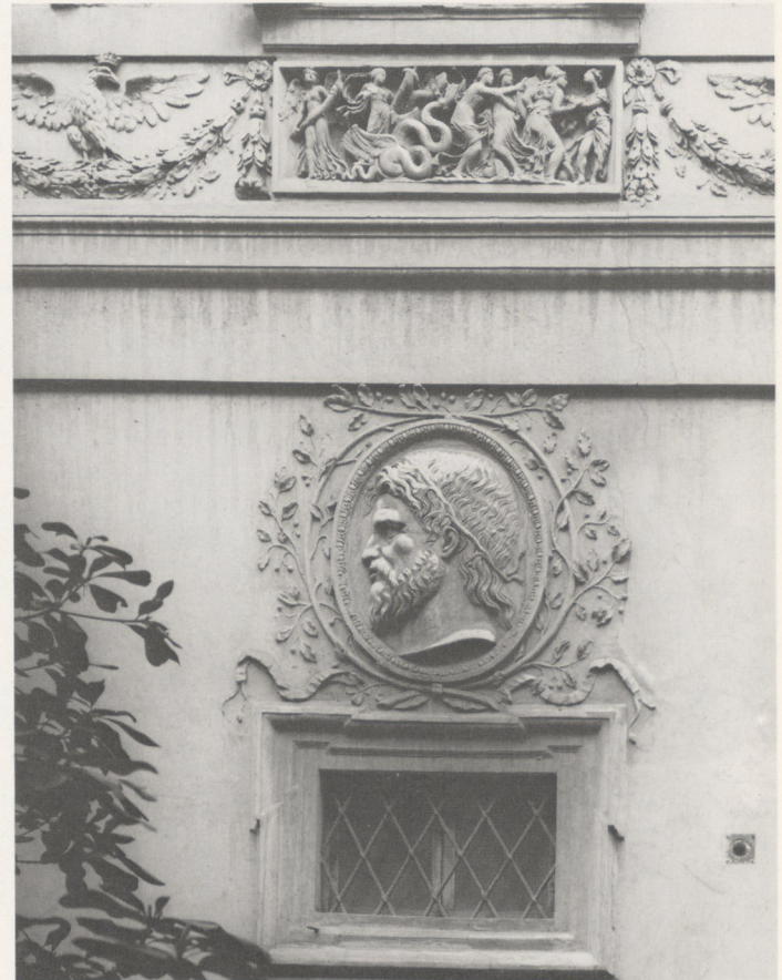
10. Casino Massimo, street facade, groundfloor and frieze
