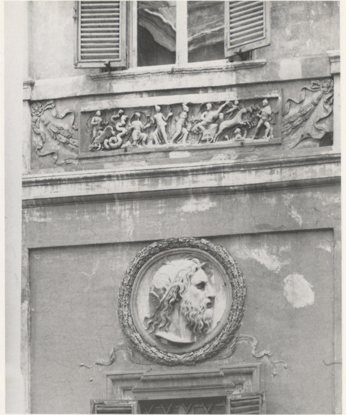
9. Casino Massimo, street facade, groundfloor and frieze
