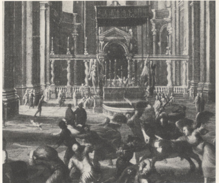
7. Detail of Fig. 6, showing 1606 baldacchino at the high altar and the ciborium with altar screen in the western apse
