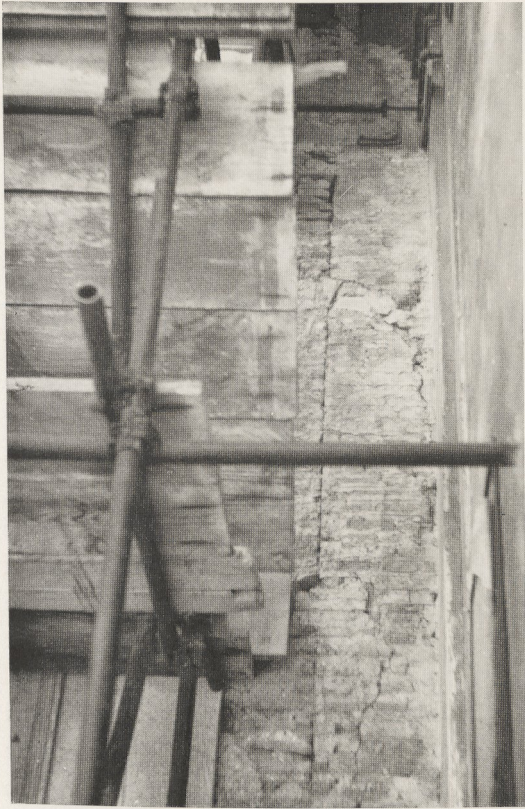
12. S. Maria in Aracoeli, vertical joint at the base of the campanile, summer 1967
