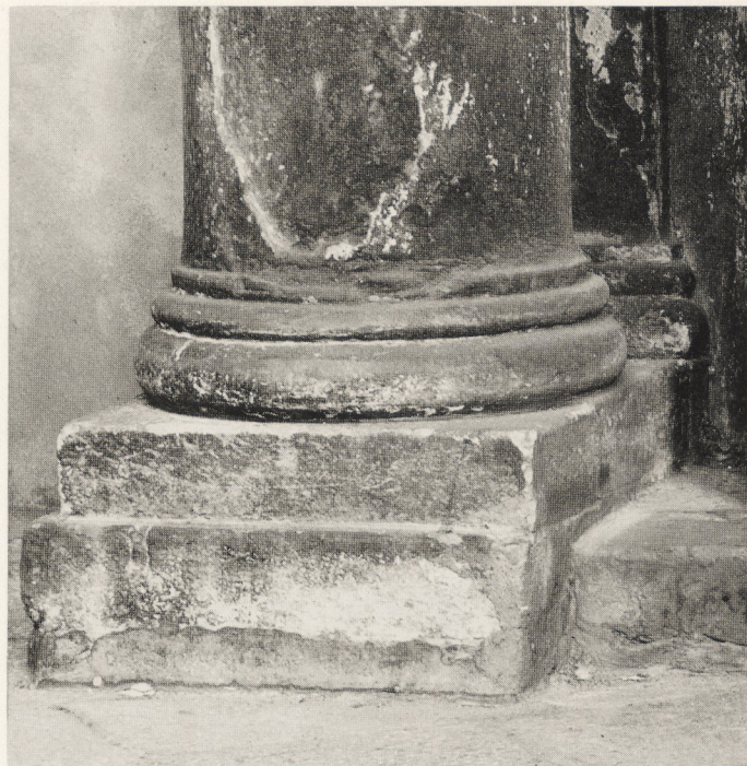
7. Doric Portal of 1547: Column base
