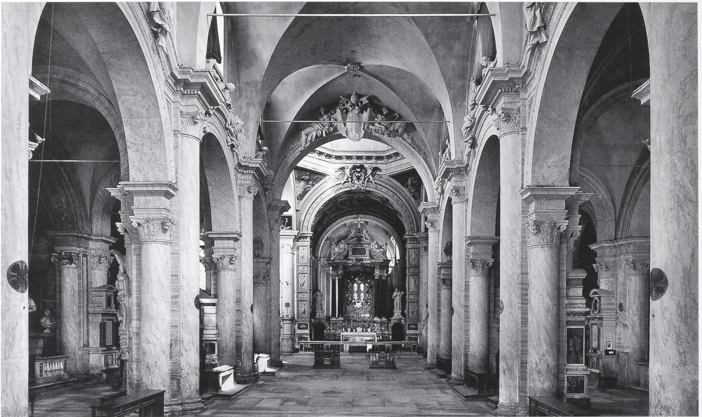
25. Gian Lorenzo Bernini, Nave Renovation. Rome, Santa Maria del Popolo
