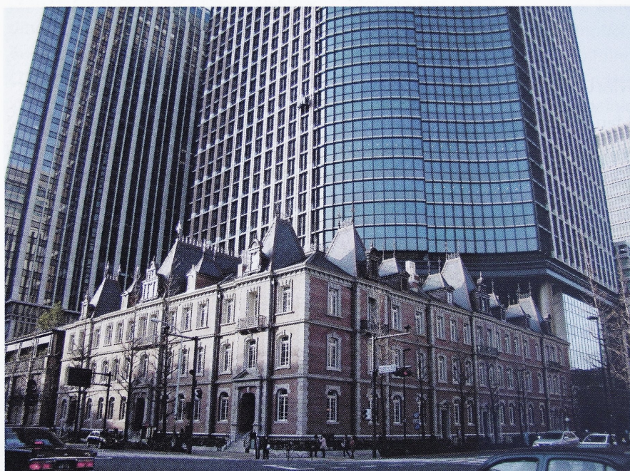
13. Marunouchi Park Building, 2009
